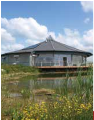
Abberton Reservoir Visitor Centre
